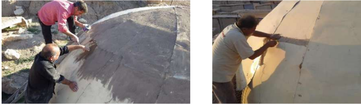
Figure 2 Showing the covering of half the dome with dirt and the experiment with burlap
