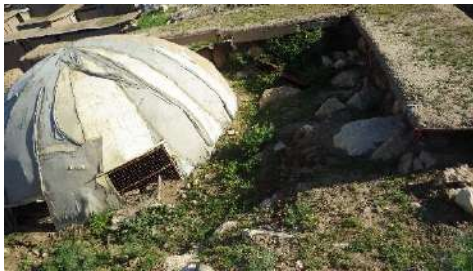
Torn burlap- Abi dome April 2016
