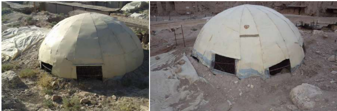
Figure 1 Photo showing the openings and the drains above the openings
