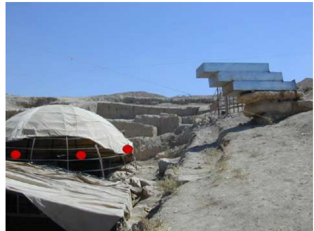
Sketches with the indication of the openings to be created in the new metal dome for aeration and light inside the Abi
