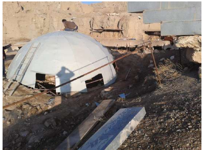
Sabah Khasseem at work (left) and detail of the openings at the base of the new Abi “dome”
